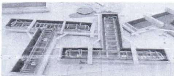
Fig. 1.9 Form work of Beam-Column joint
