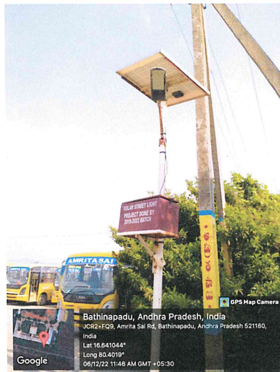
Street LED lights with Solar Panel
